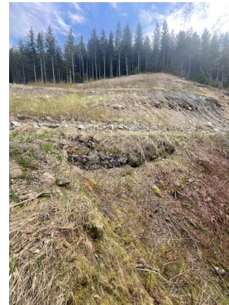
Gabions on steep foundation
